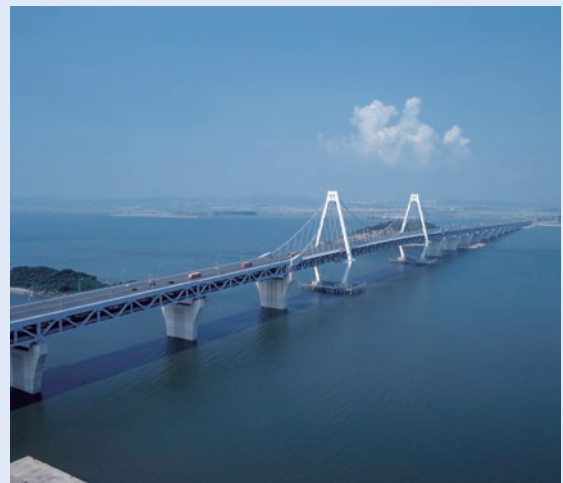
Yeongjong Grand Bridge (South Korea)
