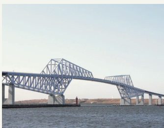
Tokyo Gate Bridge
