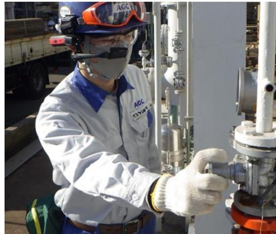
Example of operator operations using smart glasses
