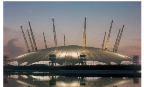
Fluon® PTFE ADs for glass cloth roofing structure (Application of weather resistance properties)
